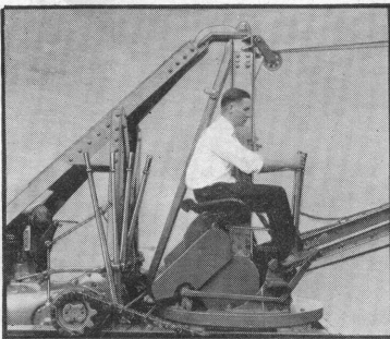
Operator in Digging Position
