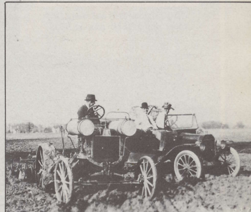
Above: Henry Ford experimented with Model T tractors from 1907 onward. Here one of the last and most improved of the flivver tractors stands alongside a conventional T. Water tanks mounted on both sides of motor. Tractor was expected to sell for $200 and was scheduled to enter the market in December 1915. But Henry Ford never offered it for sale. Below: Henry Ford's second tractor resembled a lightweight mini-steam engine complete with boiler and smokestack. The vehicle was built in the spring of 1909.
