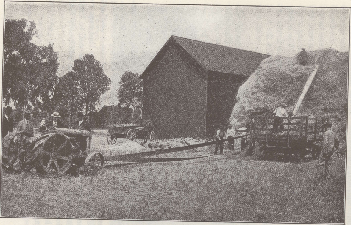
Fig. 147.—Side View Showing Method of Driving Threshing Machine by Belt Power Indicates That a Long Belt May Be Run Slack.
